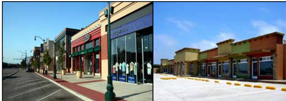
The photo on the left is an example of the recommended “town center” style development. The second photo shows a “strip mall” style development. The strip mall incorporates many elements of recommended design, but the side design still fails to create a pedestrian-oriented atmosphere.
